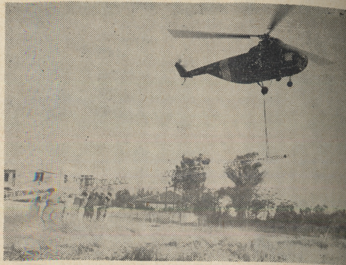
At the beginning of the lift
